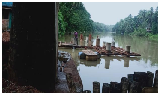
Image 5. Showing new bridge construction at Mambaram
