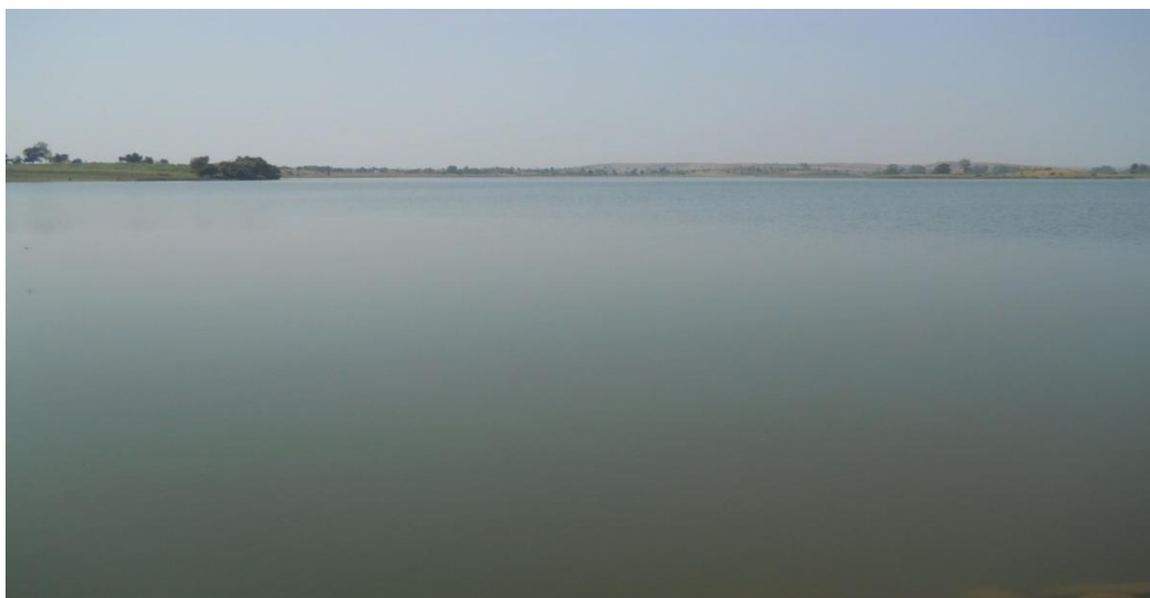
Image 2. Budki M. I. Tank –Panoramic View
